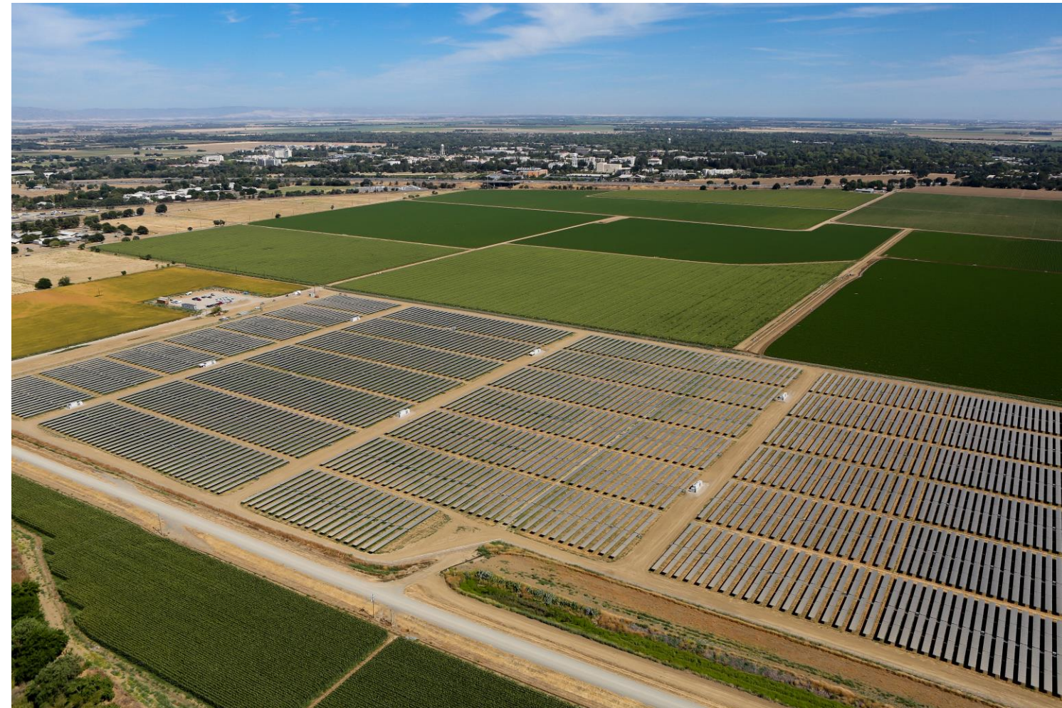
Aerial photo of UC Davis Solar Farm Looking North, July 2015 courtesy UC Davis Utilities.
