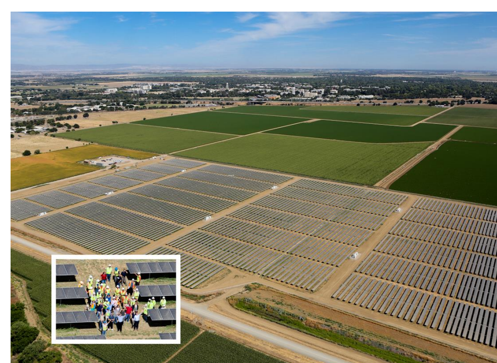
The 62 acre Sun Power solar farm on the UC Davis campus following installation of the panels. Photo taken 2015, courtesy UC Davis Utilities.
